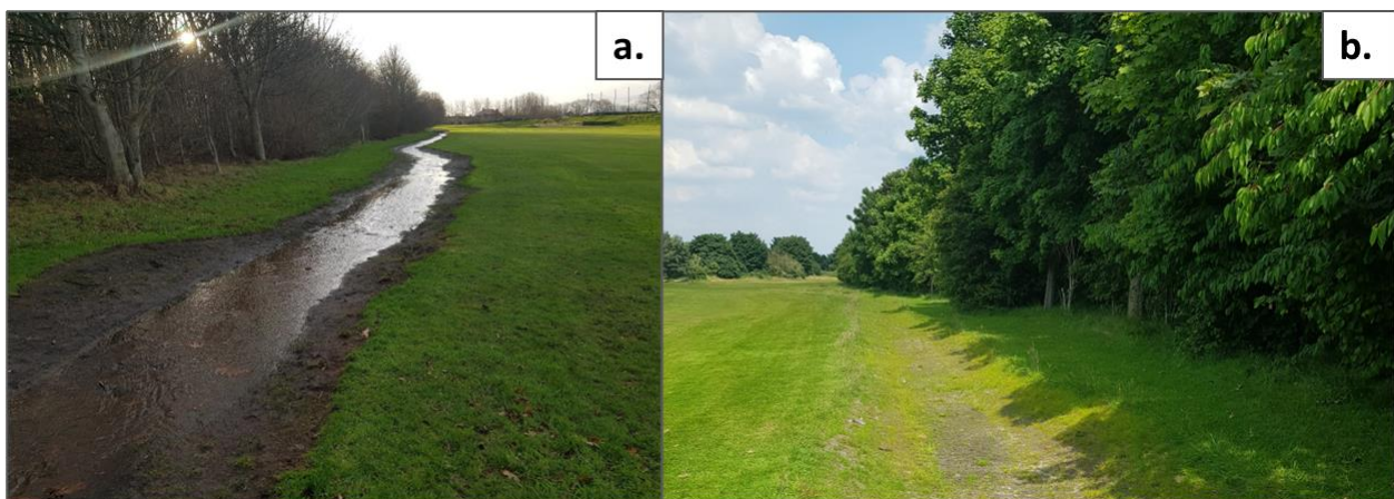
Figure 7a-b: a) Swale slowing the flow of water following heavy rain b) Vegetation beginning to become established in the swale.
